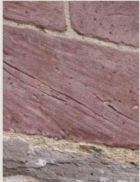
Fig. 12 Skilled contractors can achieve textures close to those in natural stone.
