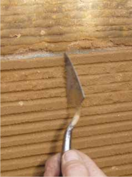
Fig. 9 Tooling of repairs should match the original stonework.
